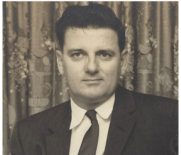
Cal Jureit who saw a way to build roof trusses that made construction scalable and housing more affordable, nearly 70 years ago.
